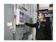
Brabazon installed a monitoring system that would maximize efficiency by turning on and off compressors to match their fluctuating demand. In addition, we are able to monitor their system remotely and alert them of any issues to maximize their uptime.
